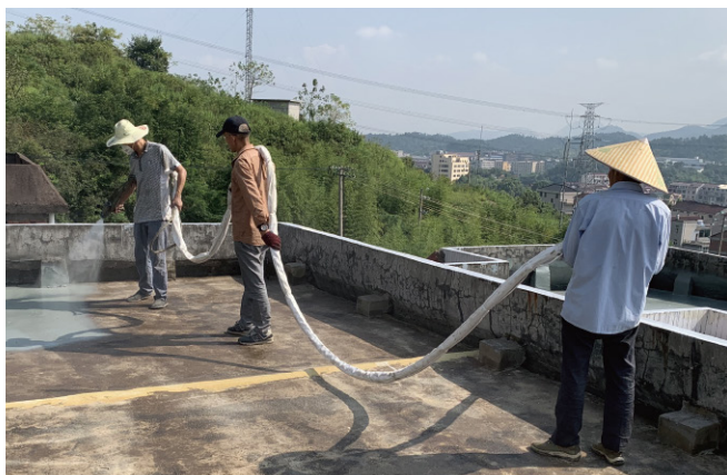
Waterproofing of flat roof
