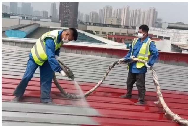
Waterproofing of sloped or inverted roof
