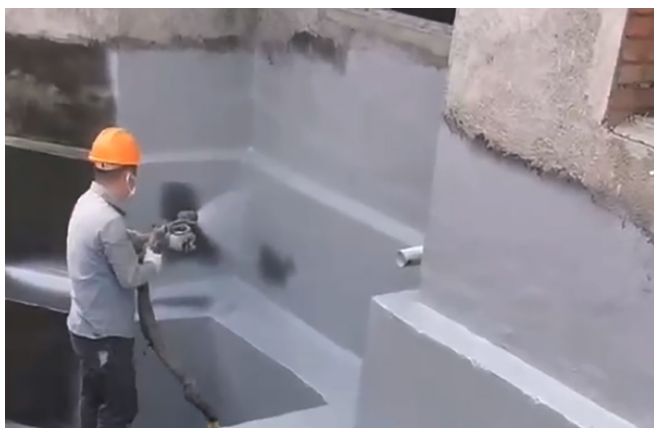
Waterproofing of Basement Exterior Wall
