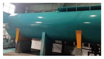
Permanent corrosion protection for both interior and exterior surfaces of industrial steel tank used to store aggressive chemicals and liquids
